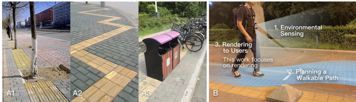
Fig. 1. (A) Examples of problems with tactile pavings: (1) obstructed by permanent constructions, (2) misused as decorations, and (3) obstructed by trash bins and bicycles. (B) The concept of Virtual Paving, a method of rendering a collision-free and smooth path to visually impaired people through non-visual feedback. This work focuses on its feedback design.
